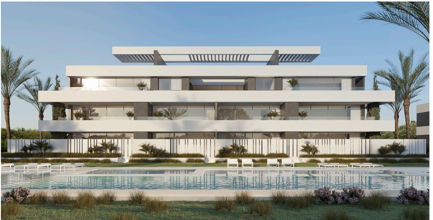
Overall view of the building's facade.
