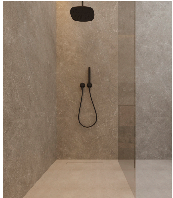
Detail of shower tray continuous with flooring
